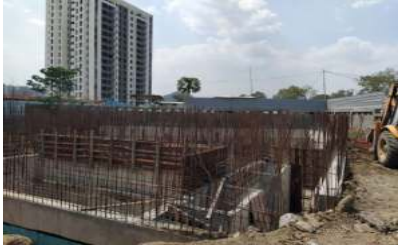
1020 KLD STP Work in Progress
